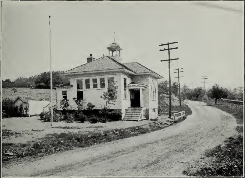
The new building in district 8, Newcastle, Westchester county
